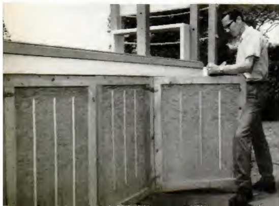
STORAGE DOORS are built with one-by stock and 1/2-in. plywood. Half-round moldings give a decorative touch
